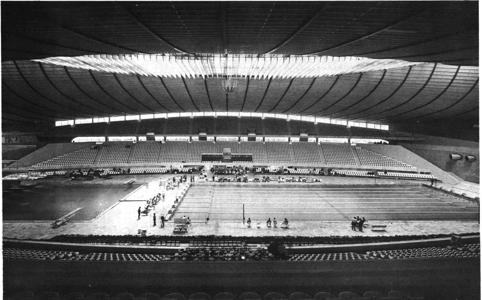
Vista interior / Interior view/(K. Miwa.)
