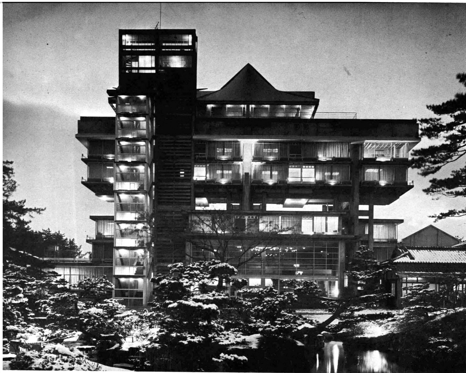
Vista general al oriente General view. East side.
