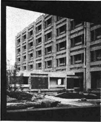
Detalle entrada / Entrance. Detail.
