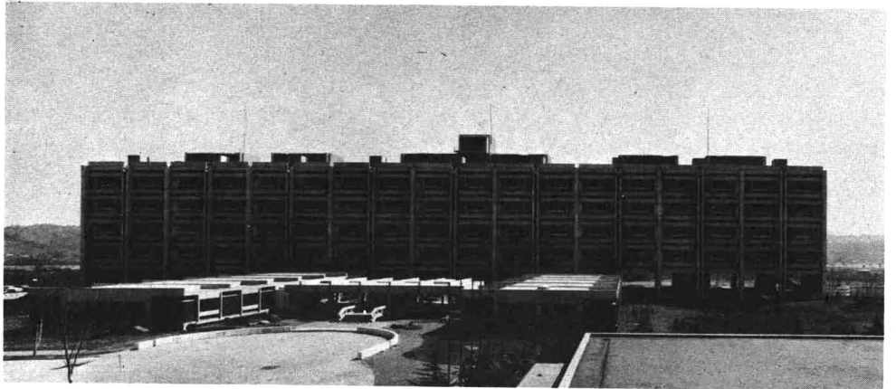
Vista general / General view.
