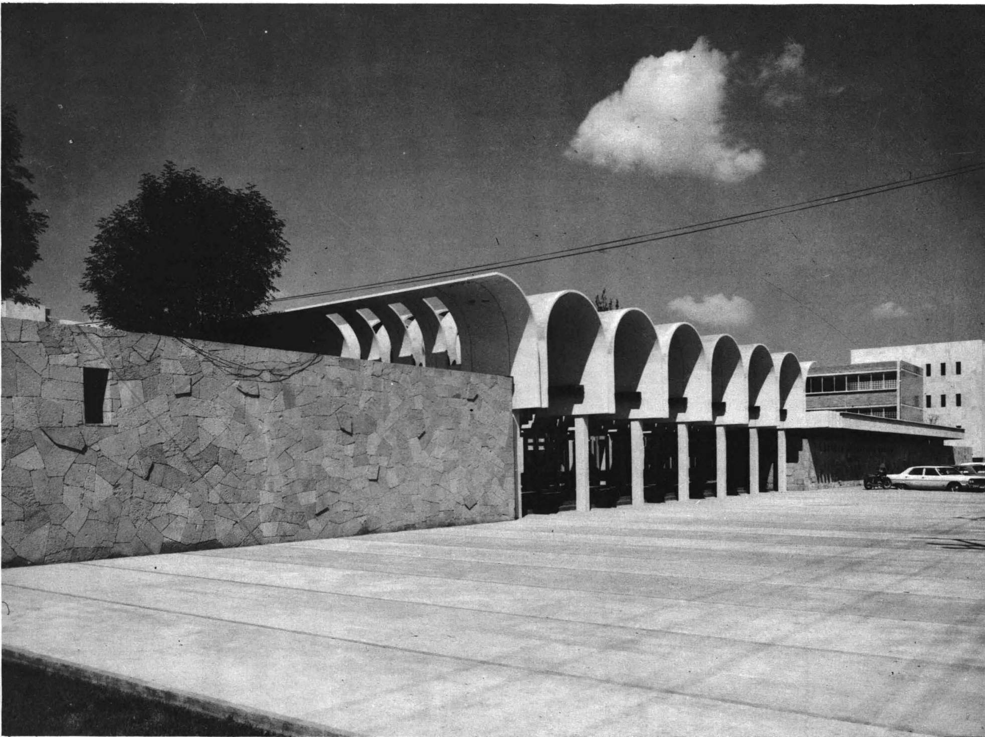
Entrada principal / Main entrance
