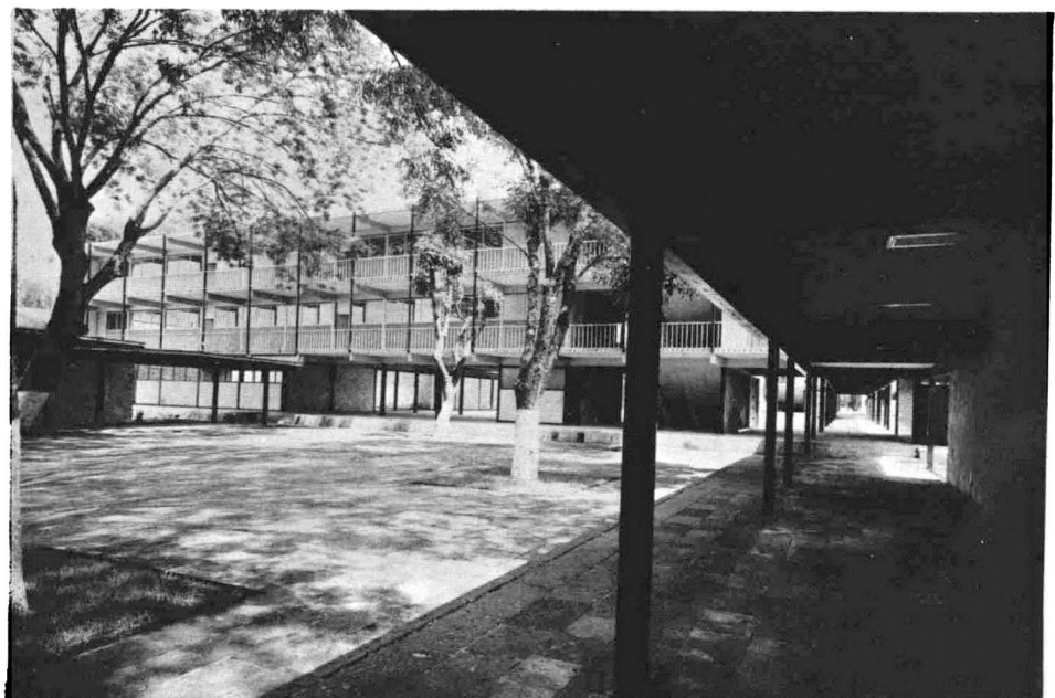
4.- Plaza and classroom buildings
